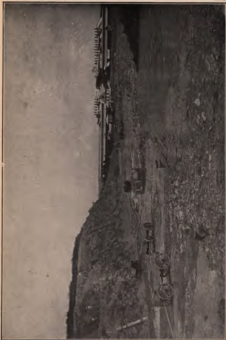
Fig. 53.— Mining Bank of Shale by Hand.
